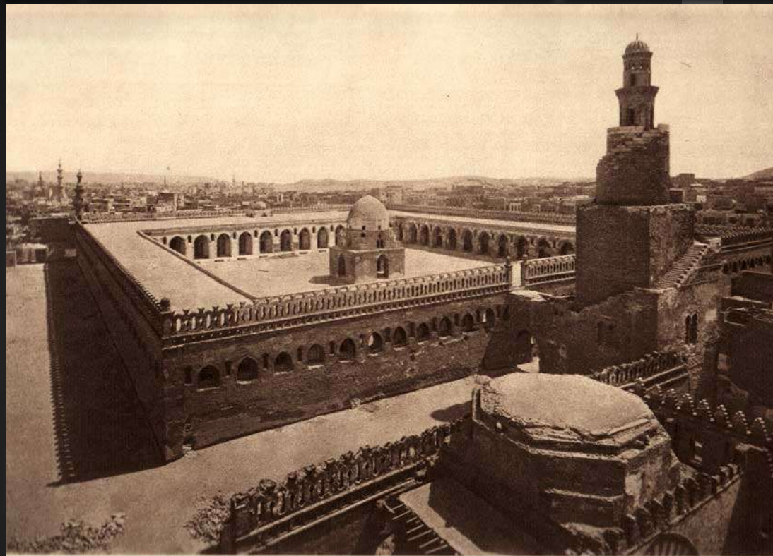
General view from the Minaret of Sarghatnuk
